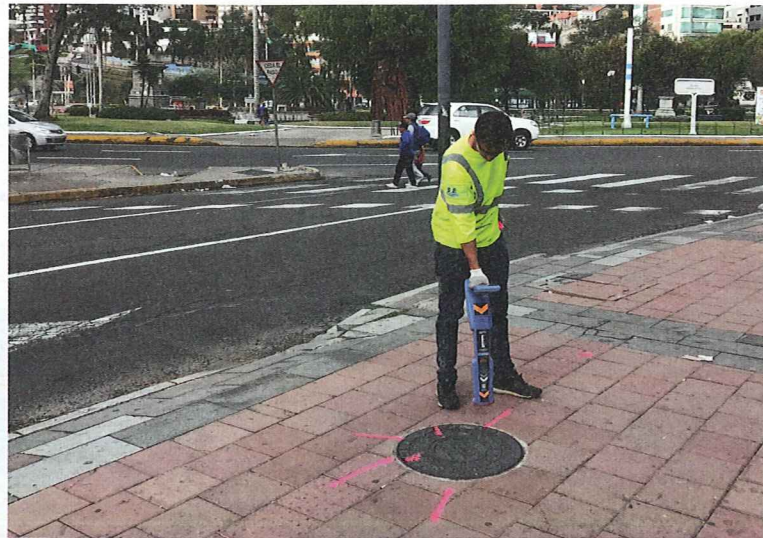
A professional SUE technician for SUE LATAM designates a line for the design phase of the Guayasamín project in Quito. As the first to use SUE in Quito, the project is a milestone for damage prevention in the nation.
